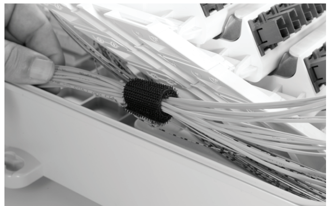
5.4 Route the pigtails to the designated adapters on the patch tray. Bundle the pigtails with hook and loop fastener when needed.
