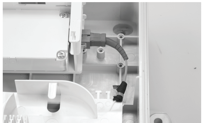
5.5 Install the incoming pigtail and route the fiber to the splicing to "splicing to splitter modules" for splicing. Remove the outer jacket over a distance of 1.2 m. Secure with foam and tie-wrap.
