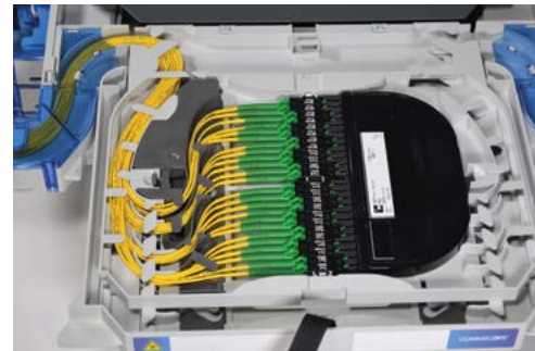
Figure 16: Value-added module shown loaded into a FACT NG4 chassis
