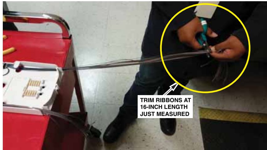
Figure 5. Trimming 1A and 1B Ribbons at 16-Inch Length
