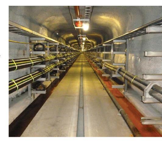
Australia's largest public utility implemented ION-M and RADIAX® radiating cable solutions from CommScope to provide seamless communication during tunnel construction.
